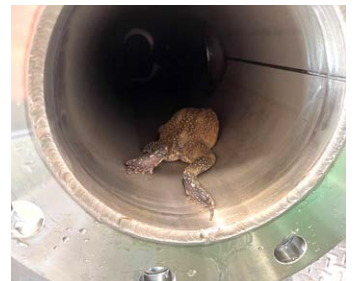
Pictured above: The pump shed was submerged, and toads caused priming problems.
