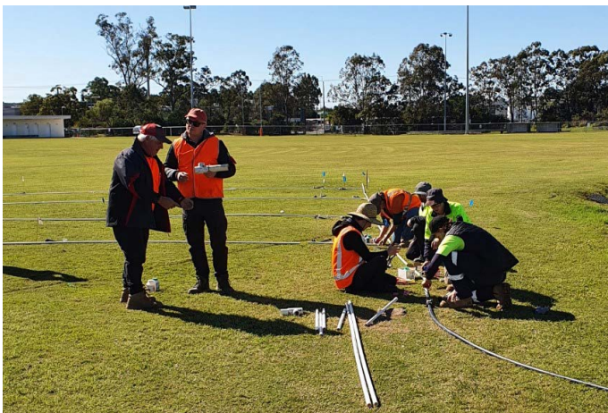
Installing a pressurised irrigation system during a training session for Certificate III in Irrigation Technology AHC32419 at Carina Leagues club (Brisbane).
